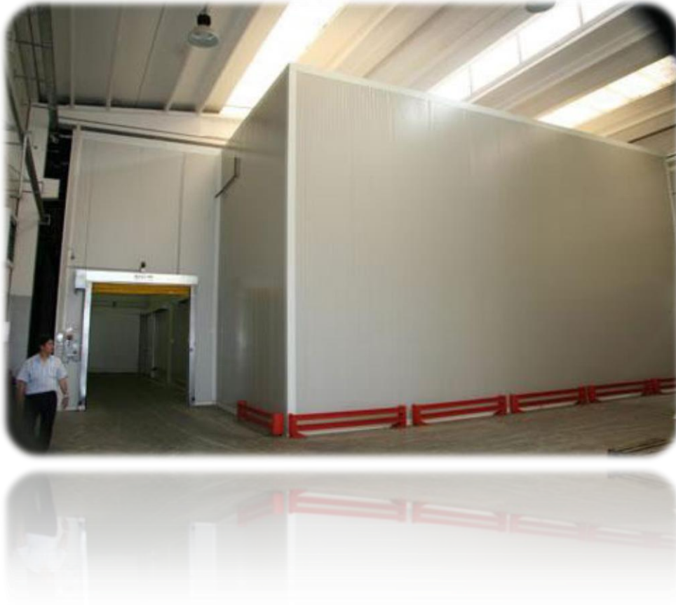
Refrigerated type ice storage room
